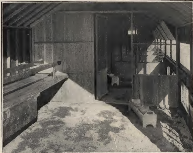
INTERIOR OF A FIVE UNIT No. 4 POULTRY HOUSE Producing perfect light and ventilation
